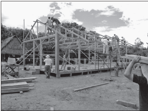
Work & Witness Church Construction in Village
